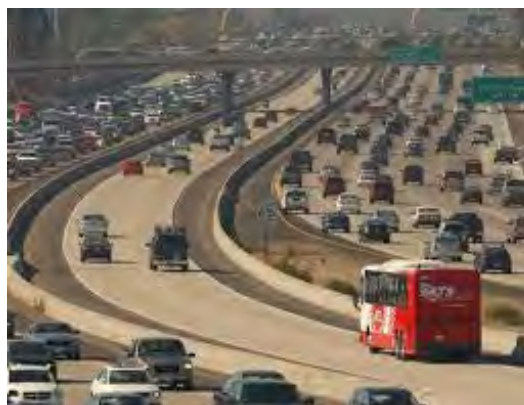
Figure 7: I-15 managed lanes (center) for HOVs, express bus service, and SOVs that pay a dynamic toll (Source: IBTTA)
